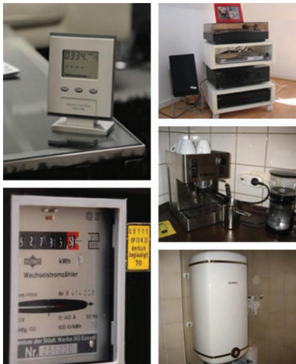
Fig. 1. A PowerMeterClock and power meter installed in one of the households (left). Some of the appliances measured by the power meter (right).
